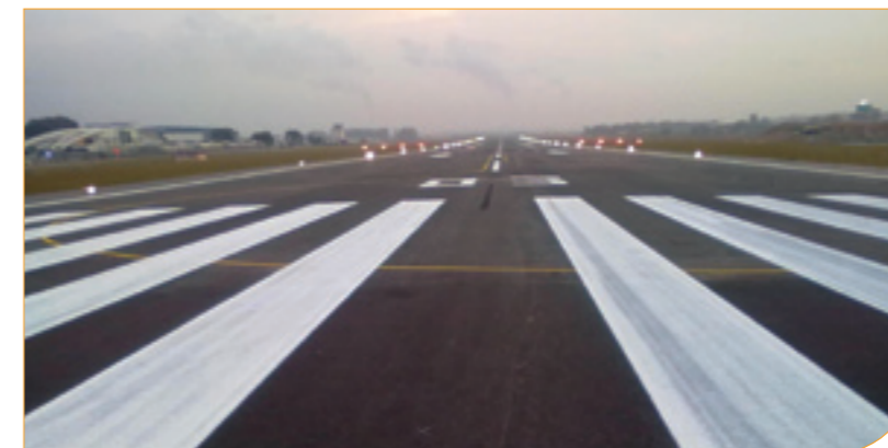
The Seletar runway was extended from 1592 metres to 1826 metres to support larger jet operations as well as heavier take-off loads expected with the growing business aviation sector.
